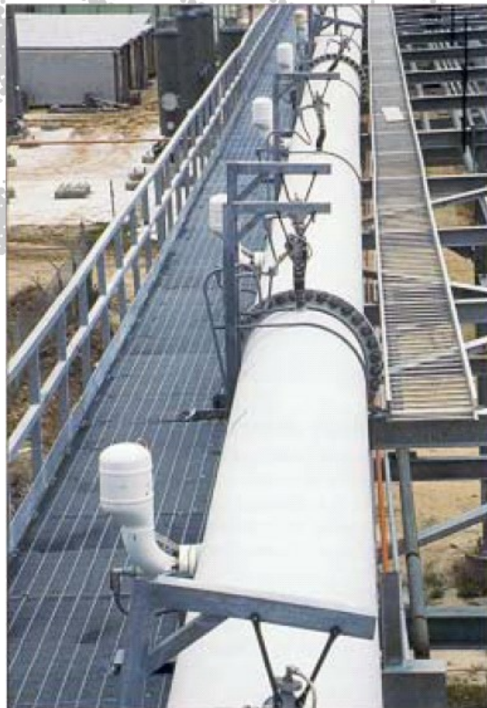
Explosion suppression system applied to pipeline
